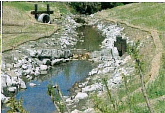
B. Cross vane grade control structure and stormwater outfall
