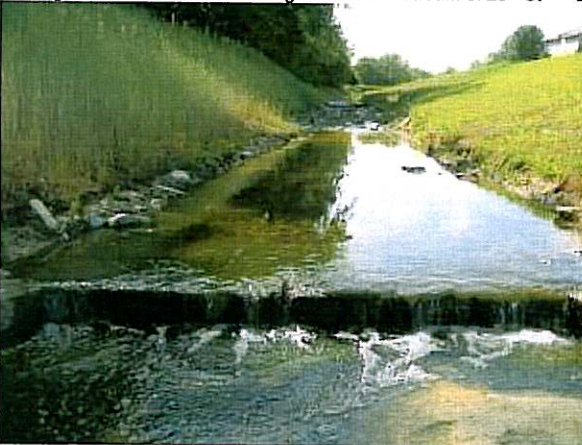
C. Series of cross vane grade control structures
